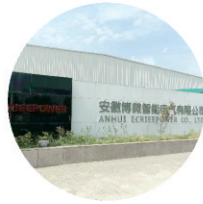
汽车电子工厂 Automotive Electronics Plant
